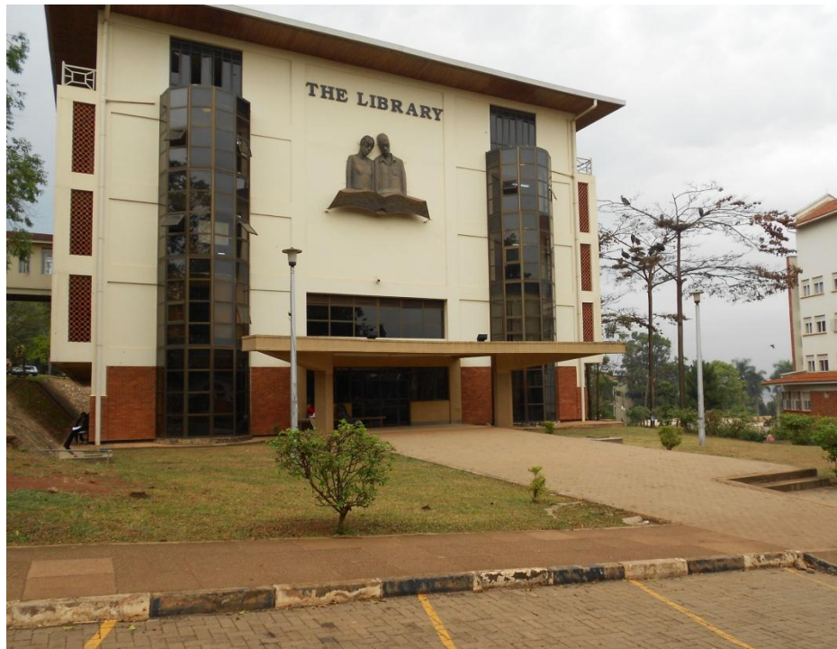
Makerere Library addition.
