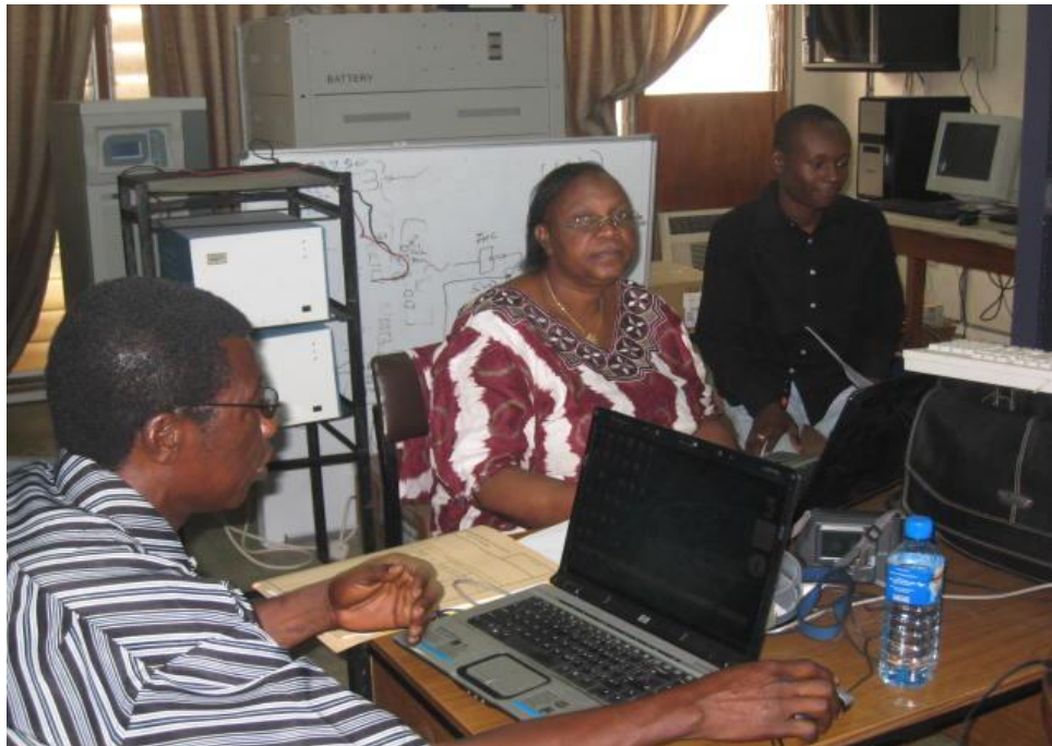
Server room and systems team at work.
